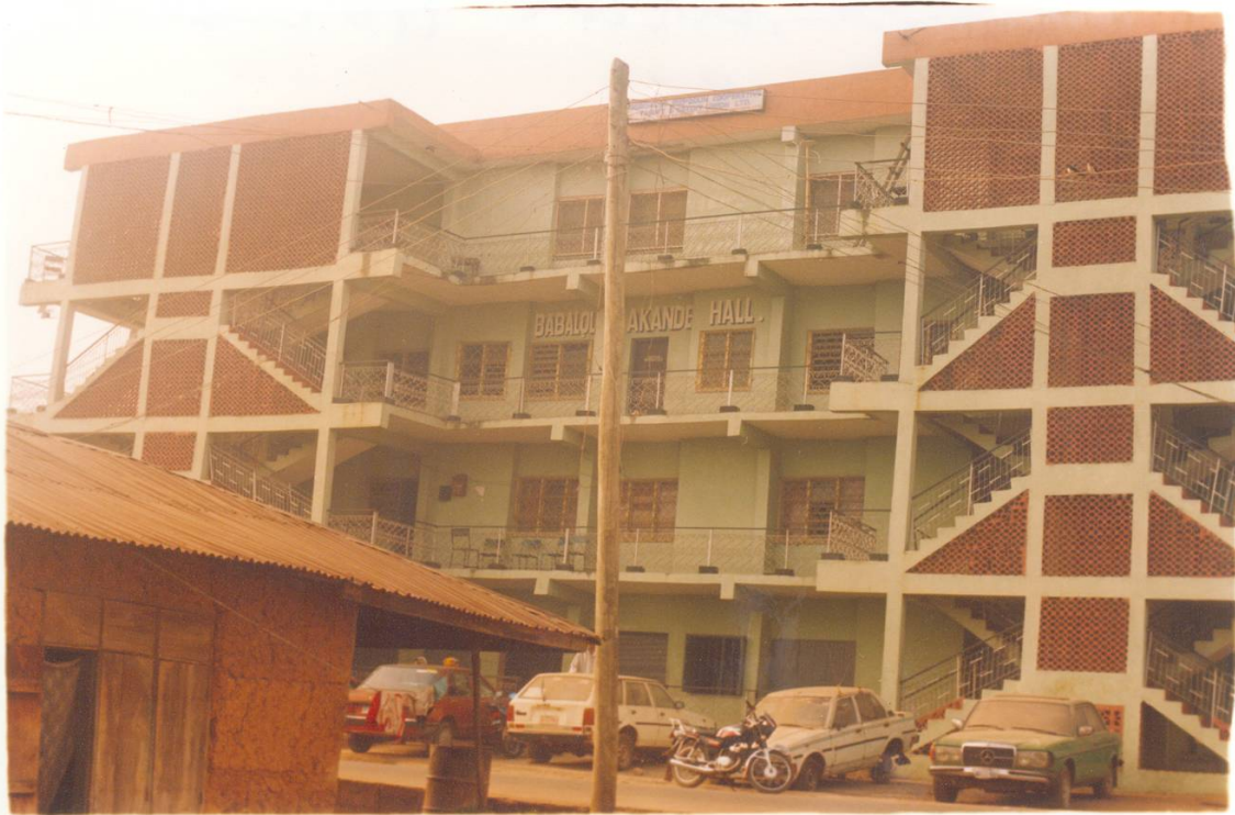
Cooperative Union Building in Ogbomosho
